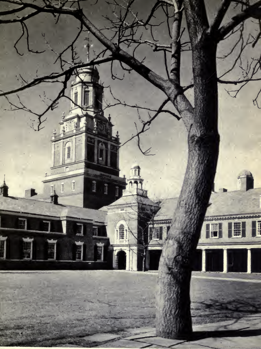
DAVENPORT COURT AND PIERSON TOWER, YALE UNIVERSITY
